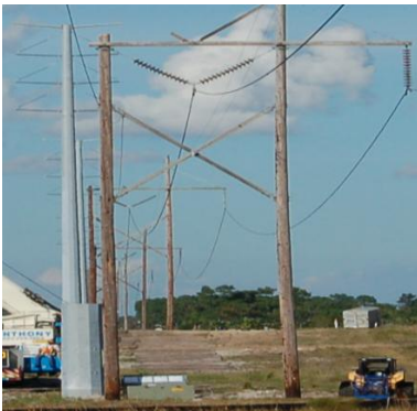
Figure 3: Visual comparison of the 230 kV single circuit, existing H-frame structure (front) and the 230 kV, double circuit, steel pole structure.
